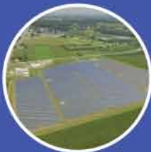
Keystone Solar Lancaster, PA
