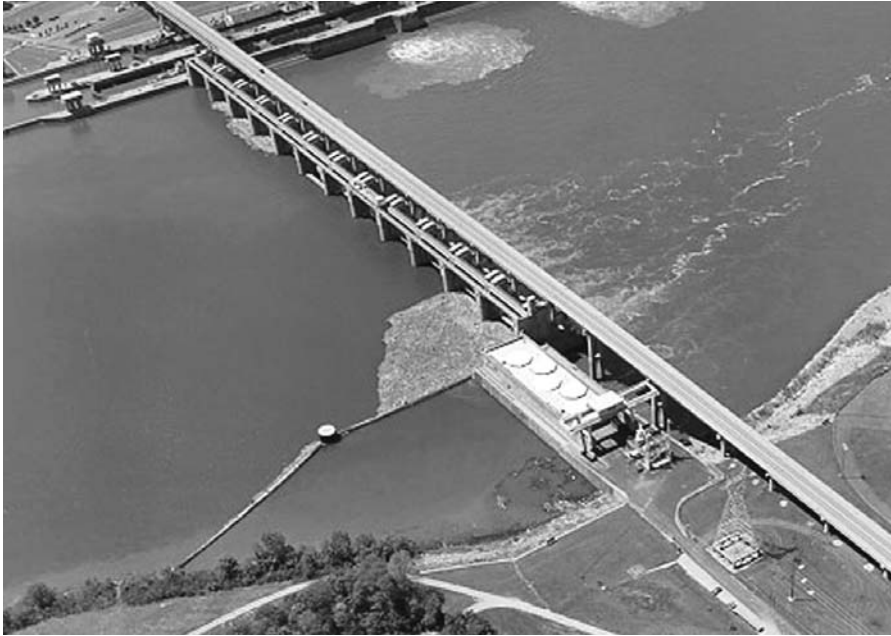
For relicensing the 64.8-MW Markland project on the Ohio River, owner Duke Energy requested and received approval from the Federal Energy Regulatory Commission to use the traditional licensing process (TLP) rather than the integrated licensing process (ILP).
